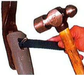
CLIP PRIOR TO INSERTION
